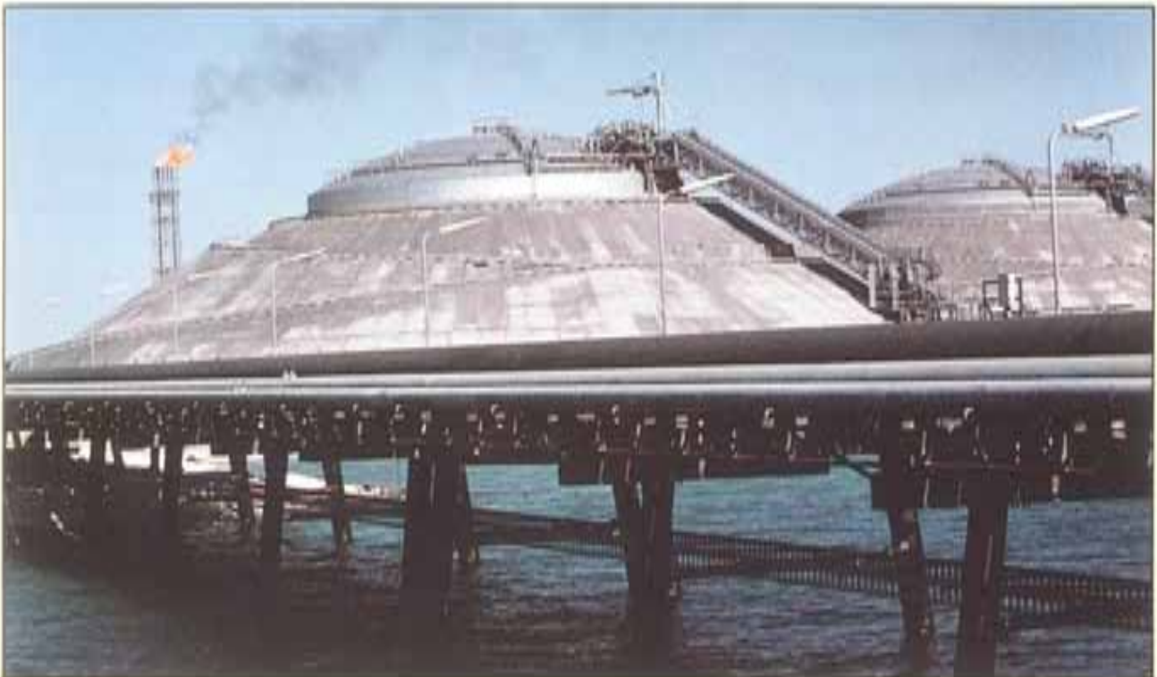
Gas Liquefaction Complex
