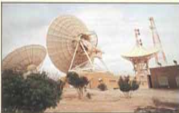
The Earth Station for Satellite Communications
